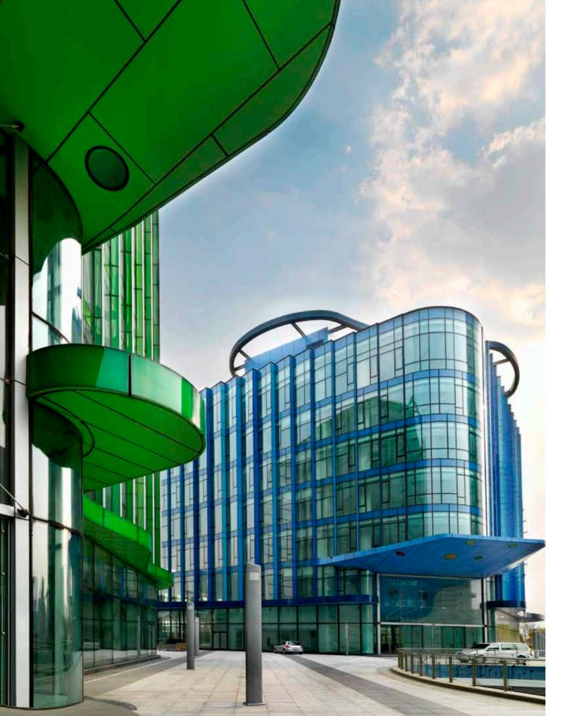
Engineered by renowned Paris-based firm RFR, the company behind the Louvre Pyramid, the facade is 12,000m<sup>2</sup> of post-tensioned glass, a visually delicate double skin that has an important environmentally sustainable role to play.
